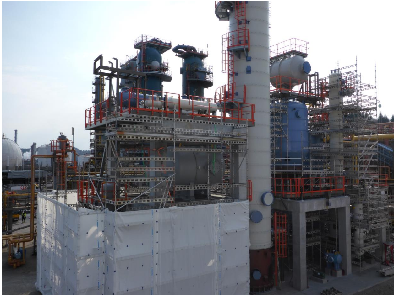
Alt mekanisk utstyr installert HTDC – April 2019
