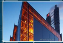
Celsio Fortum Oslo Varme AS Capture of CO 2 from waste-to-energy plant
