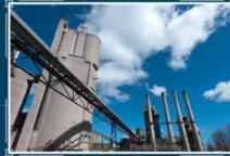
Norcem AS, Brevik Capture of CO 2 from cement plant
