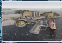
Northern Lights Intermediate storage of CO 2 onshore
